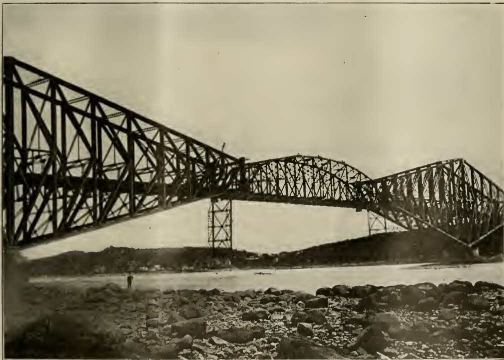
QUEBEC BRIDGE COMPLETED—CENTRAL SPAN FINALLY IN PLACE.
